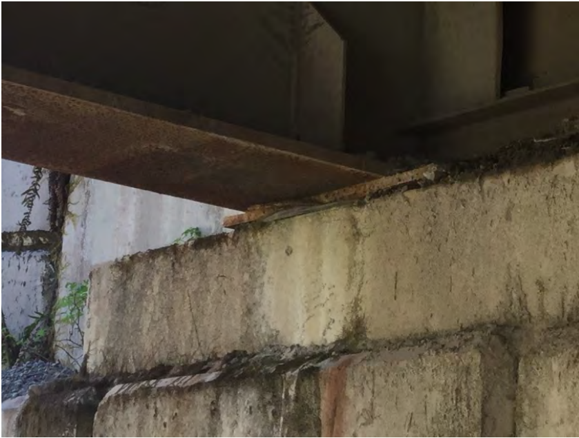
Downstream right bearing
