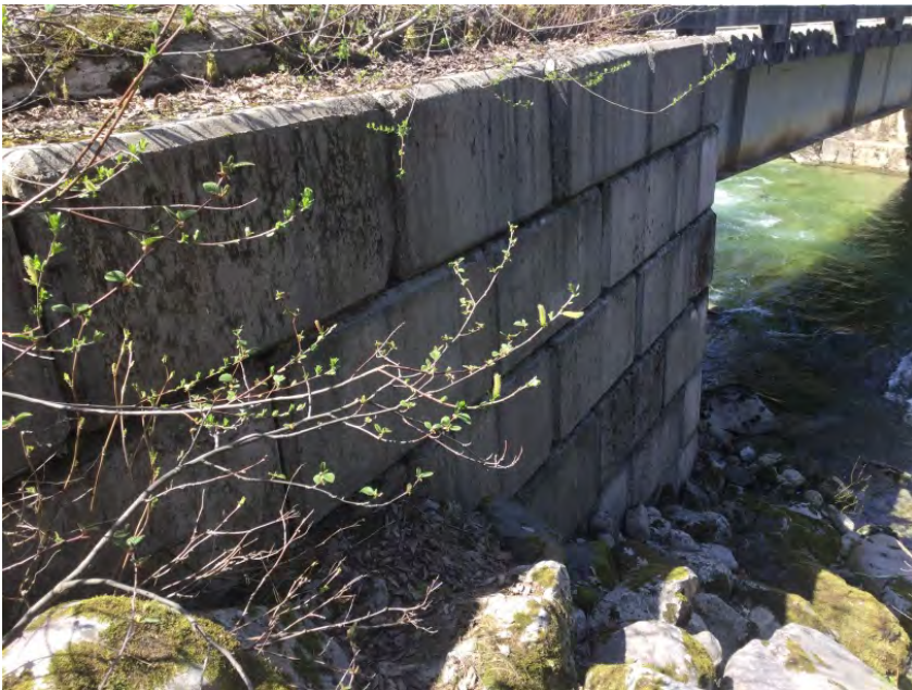
Lock block wing wall at downstream right bank
