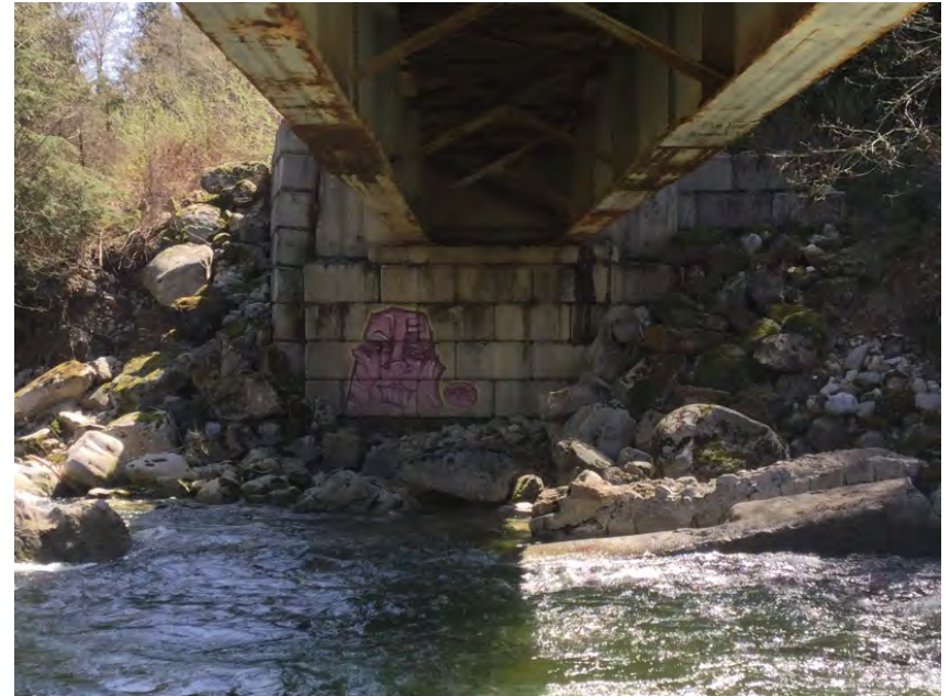
Right Bank Abutment when facing downstream
