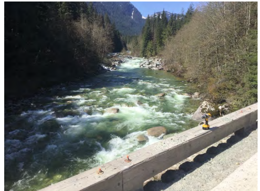
Looking upstream from deck
