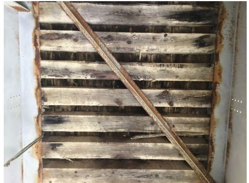
Underside of deck at left abutment
