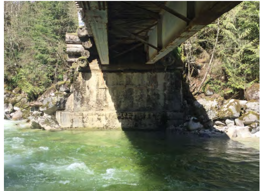
Left Bank Abutment when facing downstream
