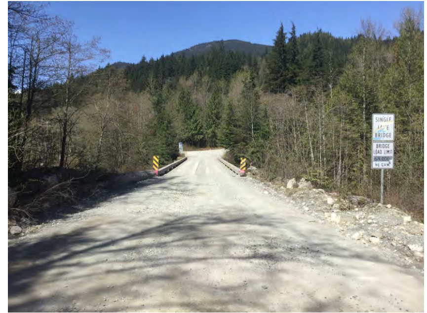
Approach from Right Bank when facing downstream
